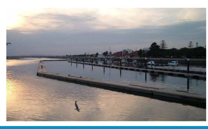
The QMF (Floating Wave Attenuator) range consists of robust, resistant and safe pontoons made of reinforced concrete with an expanded polystyrene core. Its geometry, layout, construction method and type of connections make its primary use as a wave attenuator in the protection of bays and ports.
