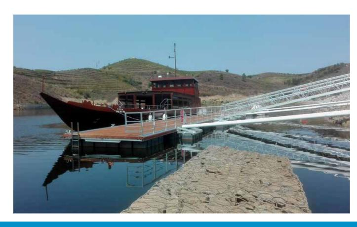
The Faro HD system consists of floating equipment with a reinforced structure in marine aluminum alloy, and is used in berthing and mooring installations of vessels in semi-enclosed bays in places with adverse environmental conditions where corrosion is a critical factor.
