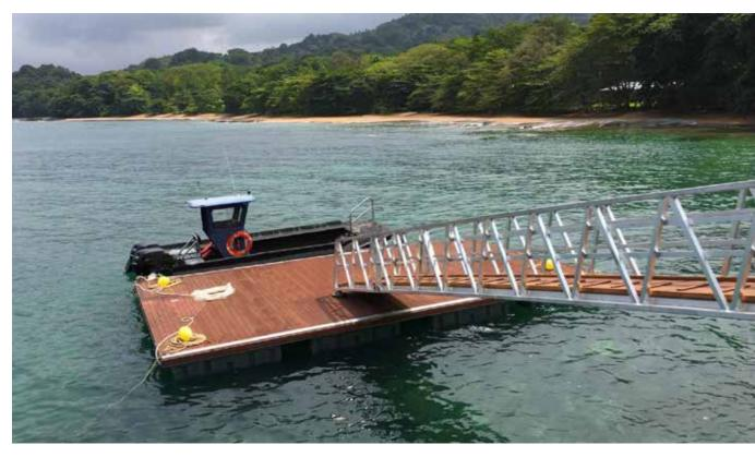
The Faro and Faro+ systems consist of floating pontoons with a special aluminum alloy profile structure composed of modular units.
