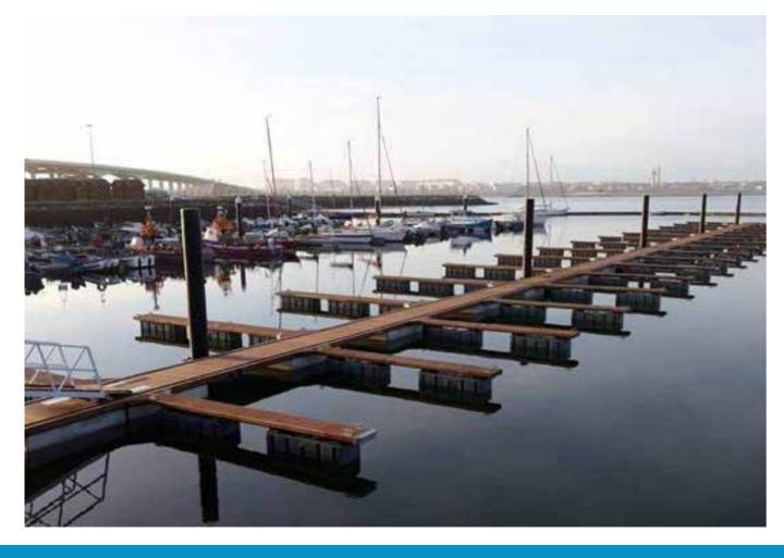
The Sagres and Sagres+ systems consist of floating pontoons with hot dip galvanized steel structure, composed of modular units and suitable for adverse weather conditions; optionally, and depending on the specific features of each application, the structures can be painted after galvanization. The walkways are supplied with ducts on both sides, covered by anodized aluminum coverings.
